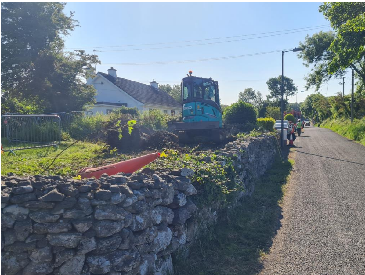
FIG.6 – ANNAGHDOWN FOOTPATH WORKS - ONGOING
