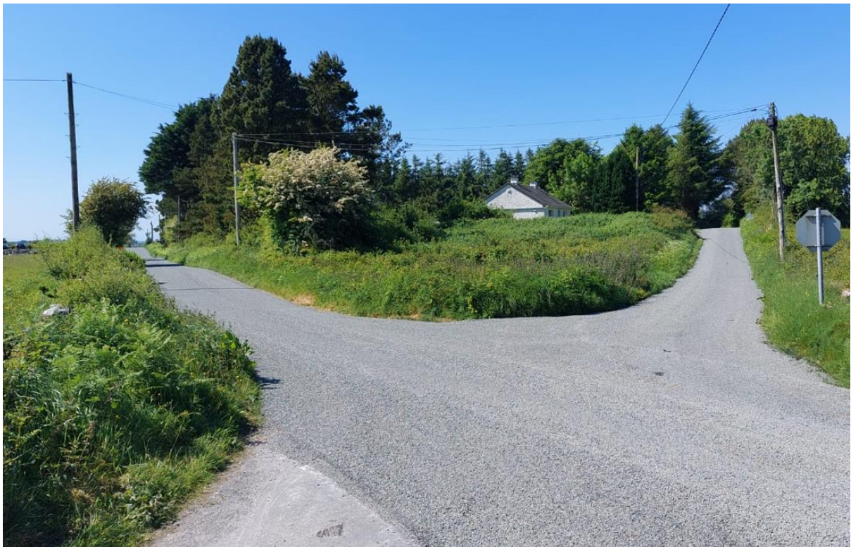
FIG.2 – FARRAVAUN SURFACE DRESSING
