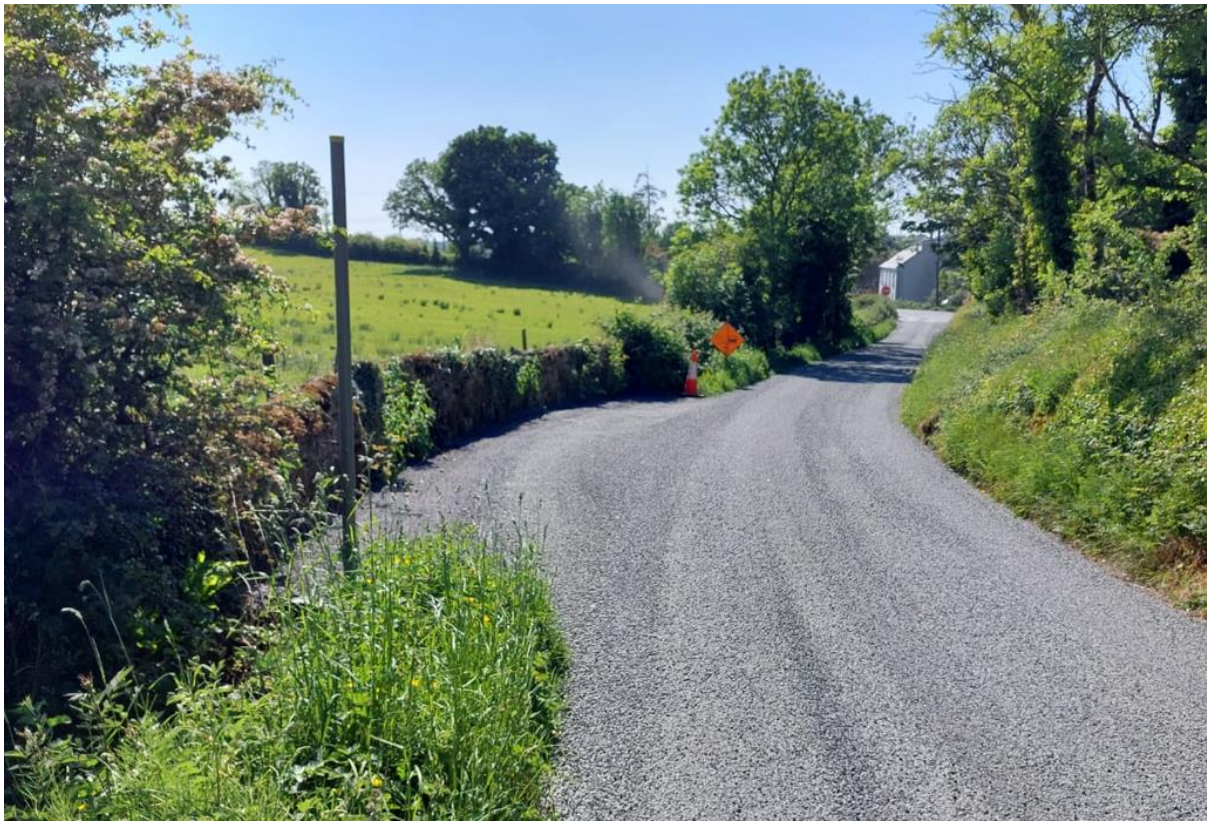
FIG.3 – GORTBRACK SURFACE DRESSING
